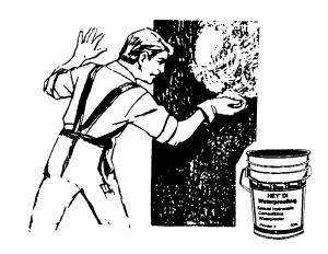
STEP 2 - As soon as the Powder X has been applied, brush the area with Hey'di sealing liquid using a clean brush.
