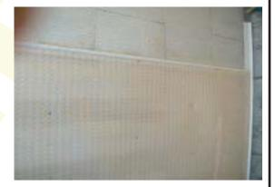
The Dimpled Sheet is resistant to a wide range of chemicals, resistant to fungus and bacterial attack, impervious to root penetration and rot proof.
