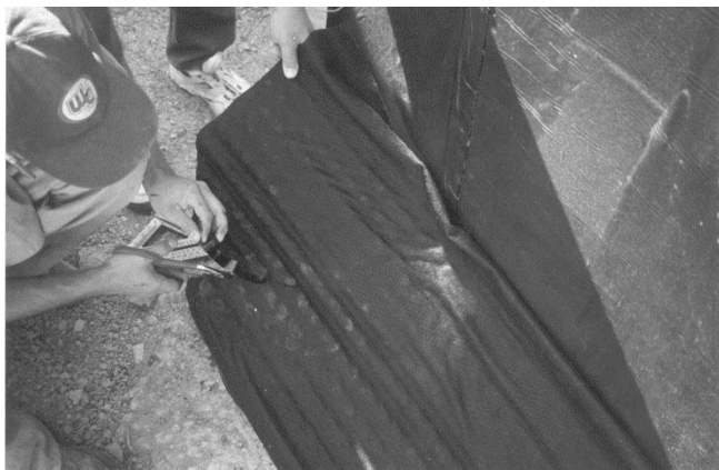
CCW QuickDRAIN being fitted for a corner
